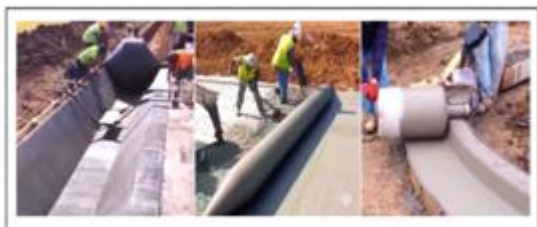
Figure 1. Road, sidewalk, irrigation and waterways technology [29]
