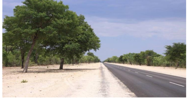
Figure 1: Road upgrade Ohangwena Region
